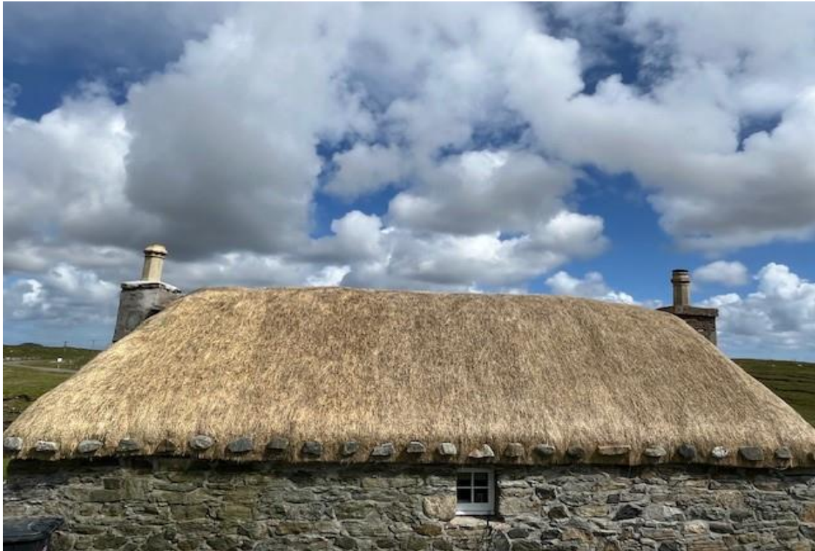
Photograph of back of thatched property. Photo Credit: Esther MacDonald
