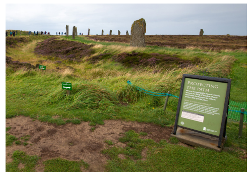
Top: Maintenance at Edinburgh Castle Middle: Soft capping at Melrose Abbey Bottom: Visitor management to protect the Ring of Brodgar from the erosion caused by high footfall and weather.
