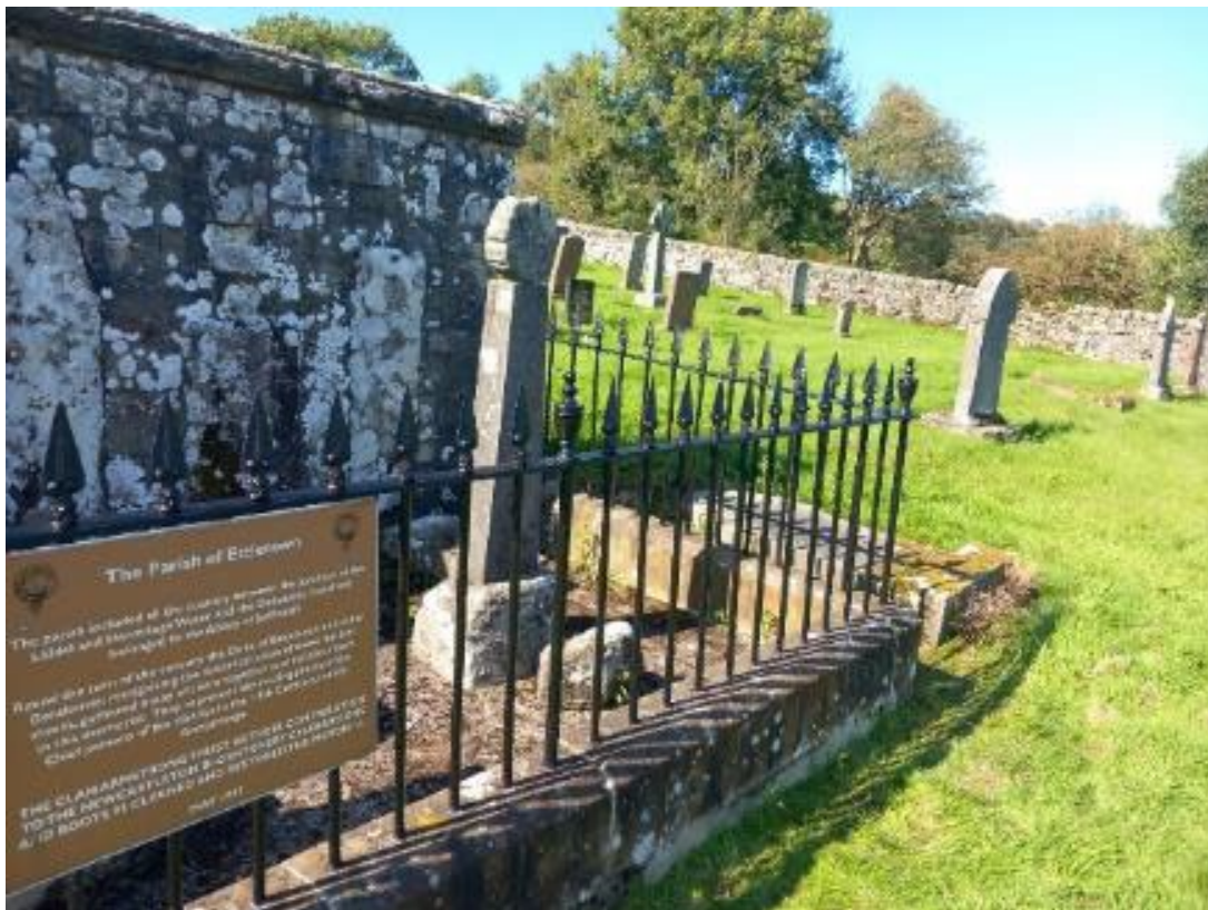
Figure 16 Completed works showing the repaired enclosure
