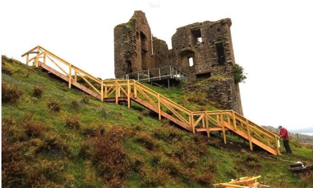
Figure 11 Maintenance of pathways and stairs to allow public access to the monument
