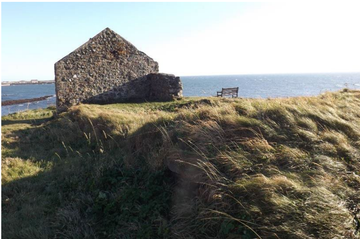
Figure 10 View of the chapel after strimming
