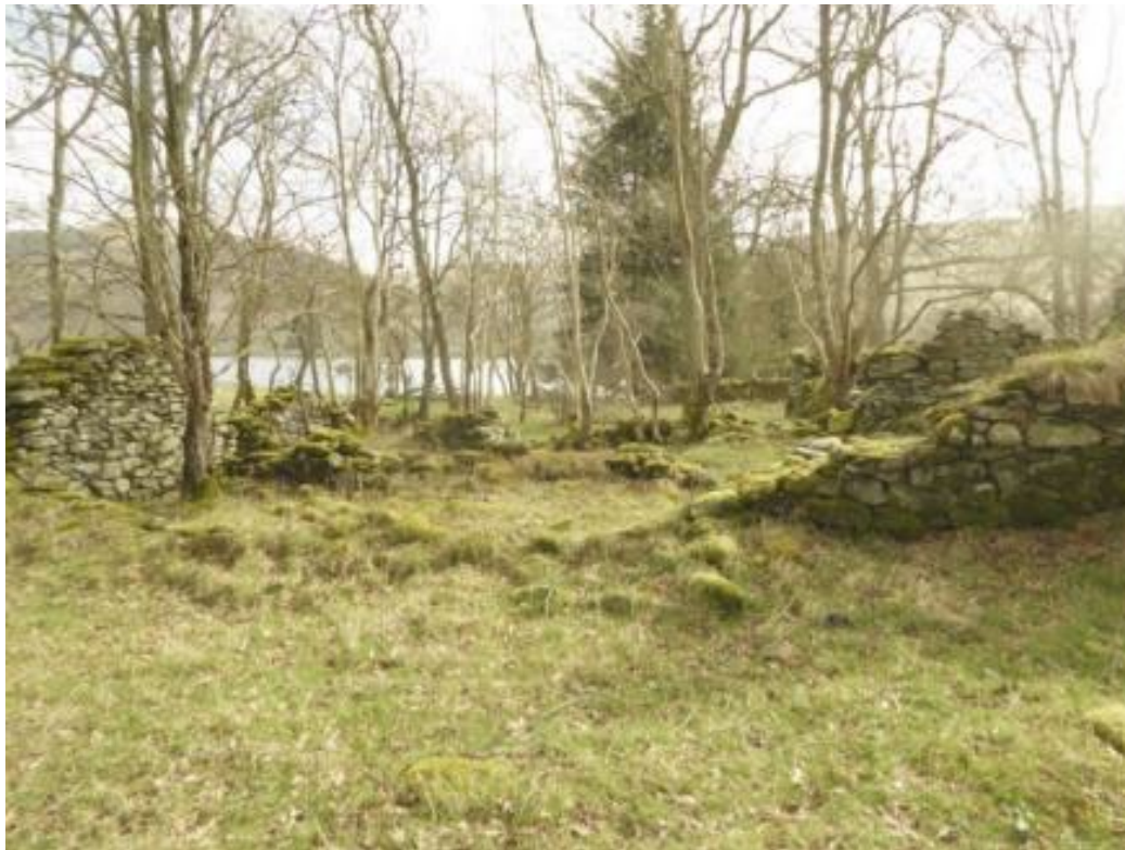
Figure 7 View of the building remains prior to works commencing
