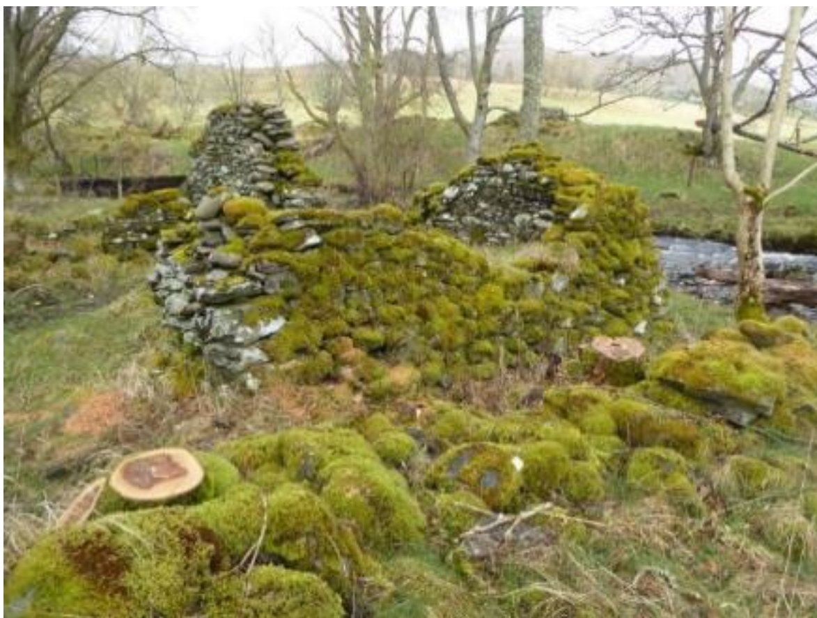
Figure 8 View of the monument with trees removed and stumps treated
