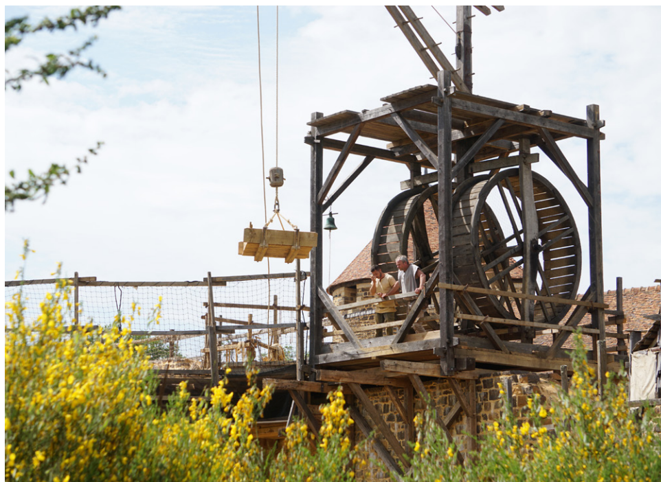
A treadwheel crane in use at Castle Guedelon.
