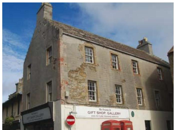
Failure of a render and associated stone decay caused by the use of incompatible cement based mortar.
