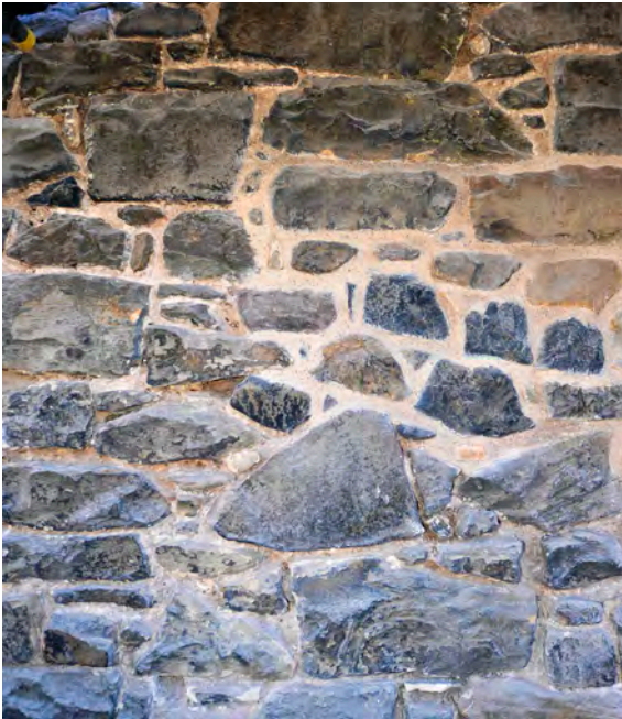
Mortar pointing, Edinburgh Castle
