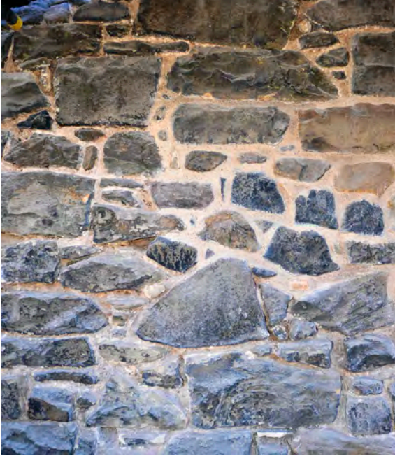
Mortar pointing, Edinburgh Castle
