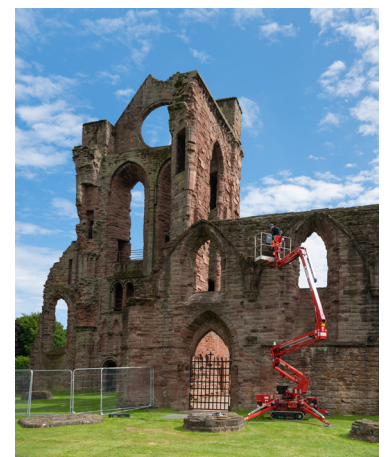
High level masonry inspection, Arbroath Abbey.
